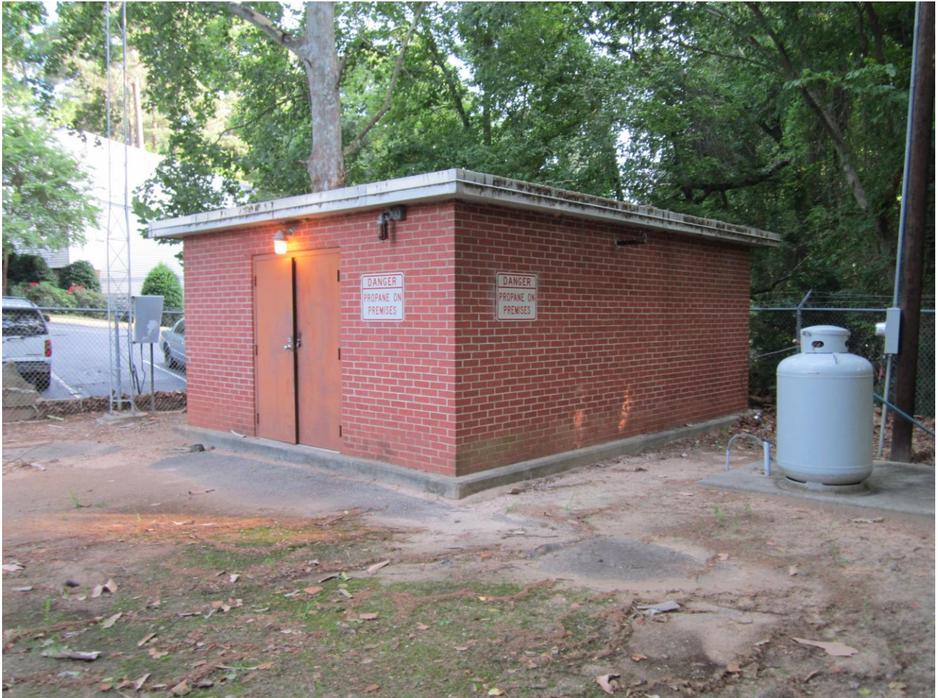
PHOTO 1: OVERALL PUMP STATION SITE
