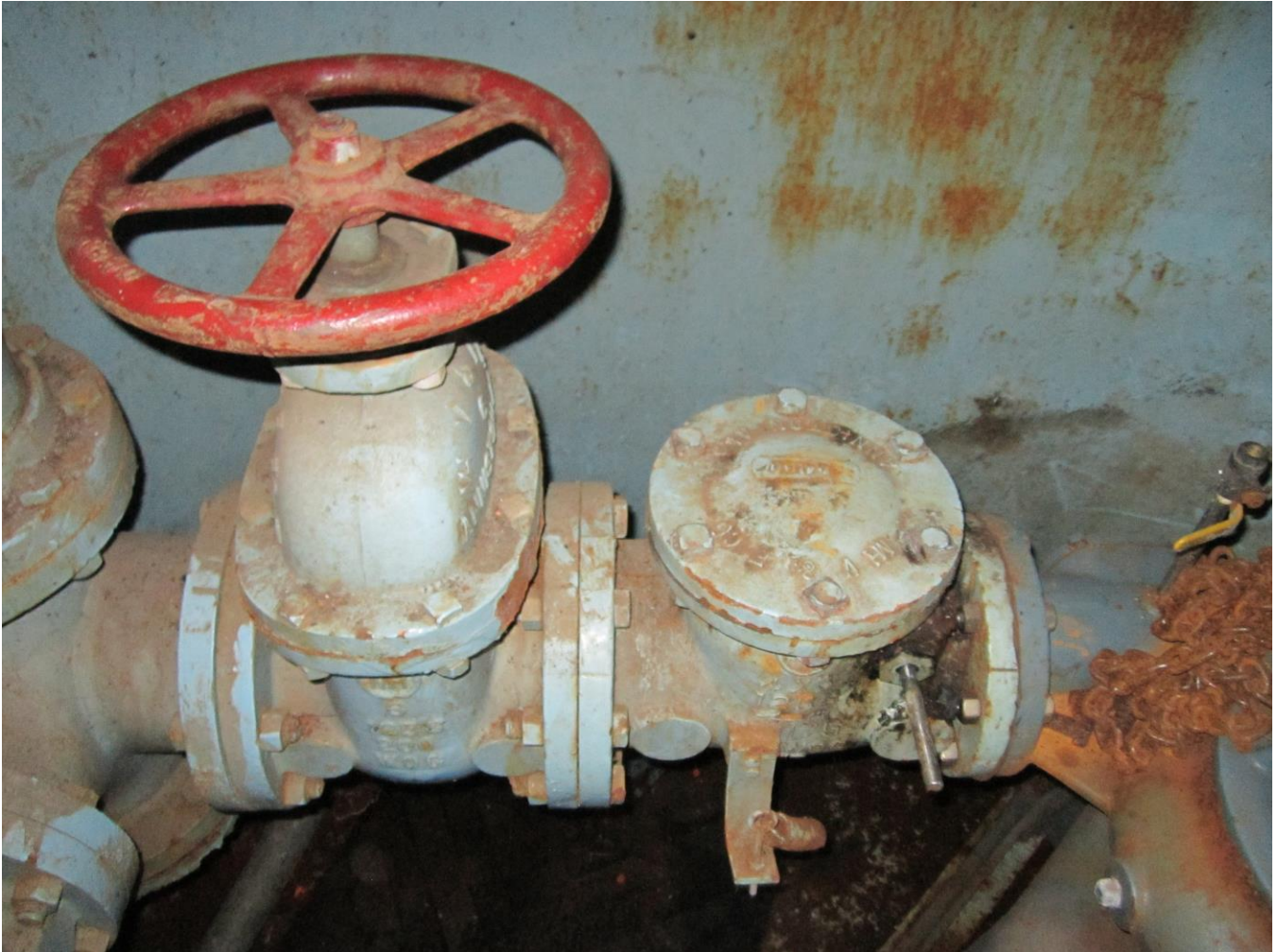
PHOTO 2: DISCHARGE HEADER
