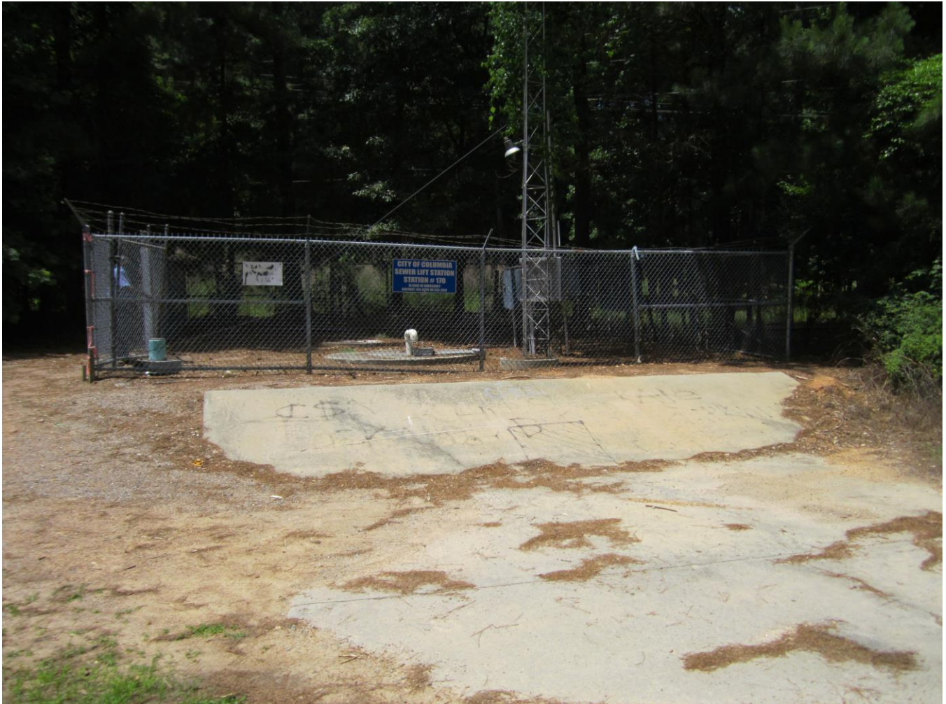
PHOTO 1: OVERALL PUMP STATION SITE AND ENTRANCE
