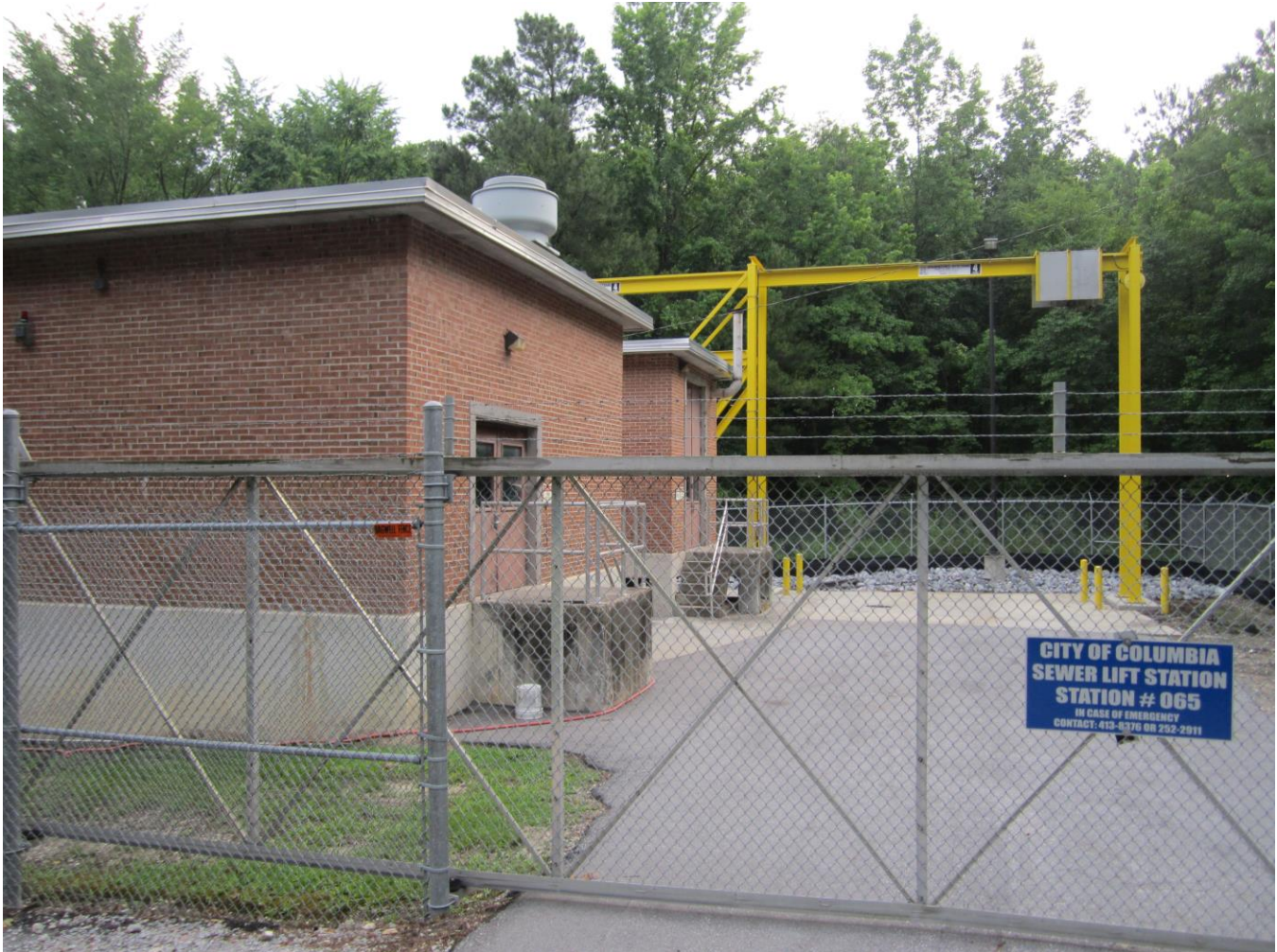
PHOTO 1: OVERALL PUMP STATION AND SITE ENTRANCE
