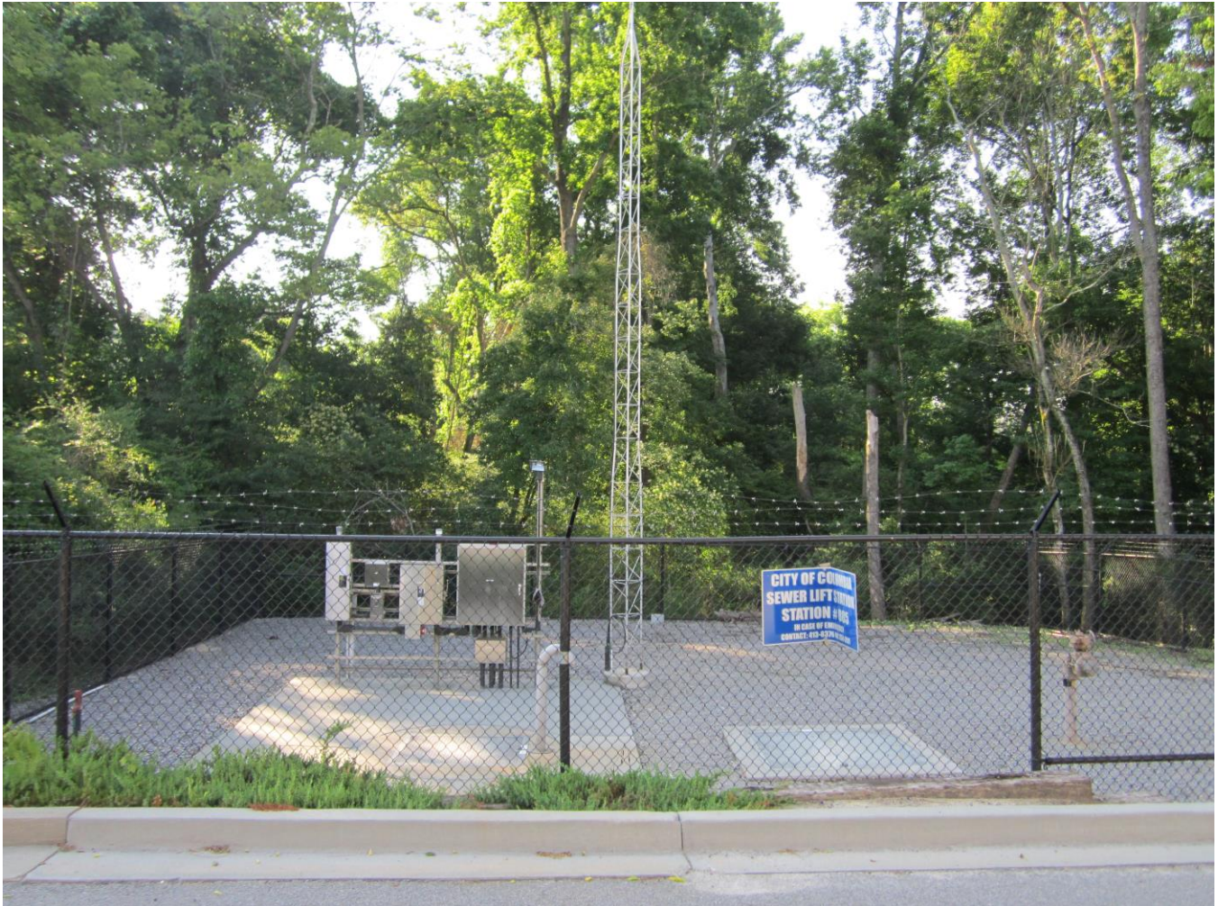
PHOTO 1: OVERALL PUMP STATION AND SITE ENTRANCE
