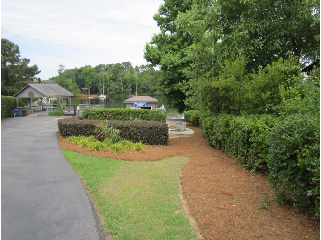
PHOTO 1: OVERALL PUMP STATION SITE
