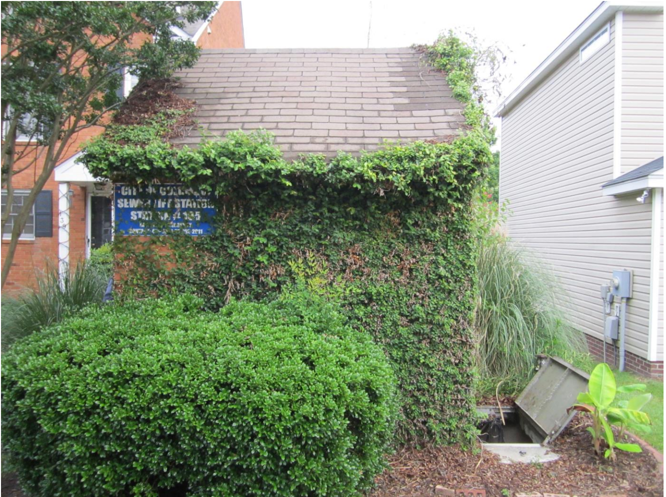
PHOTO 1: PUMP STATION EXTERIOR
