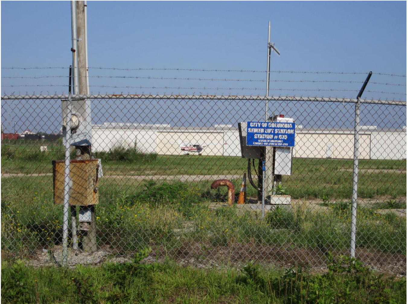
PHOTO 1: OVERALL PUMP STATION SITE
