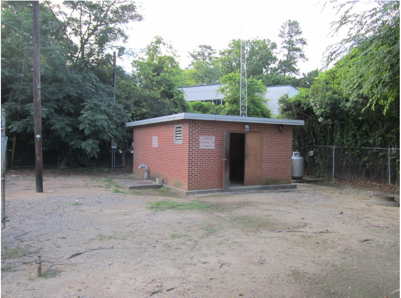
PHOTO 1: OVERALL PUMP STATION SITE AND ENTRANCE
