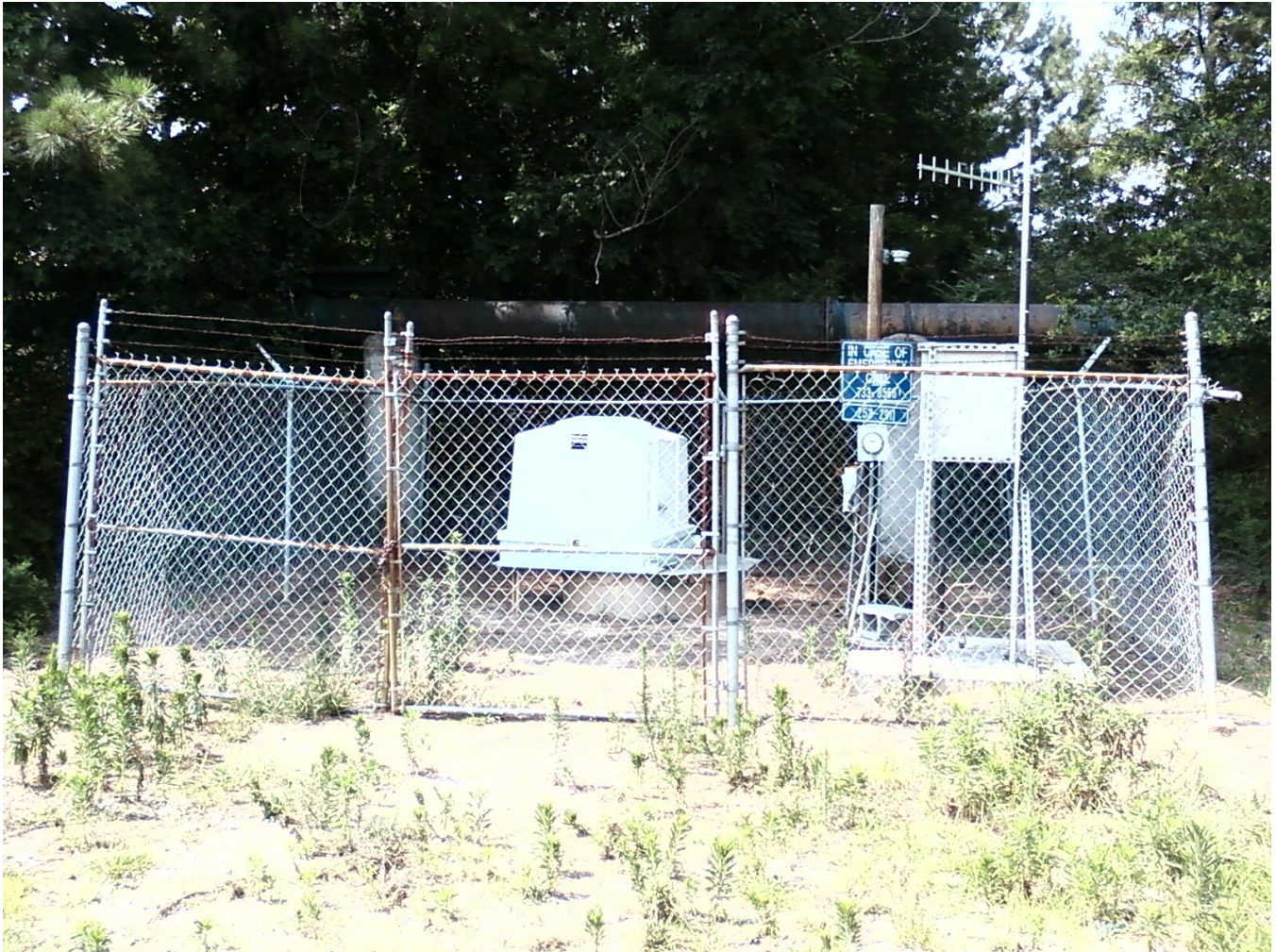
PHOTO 1: OVERALL PUMP STATION SITE AND ENTRANCE
