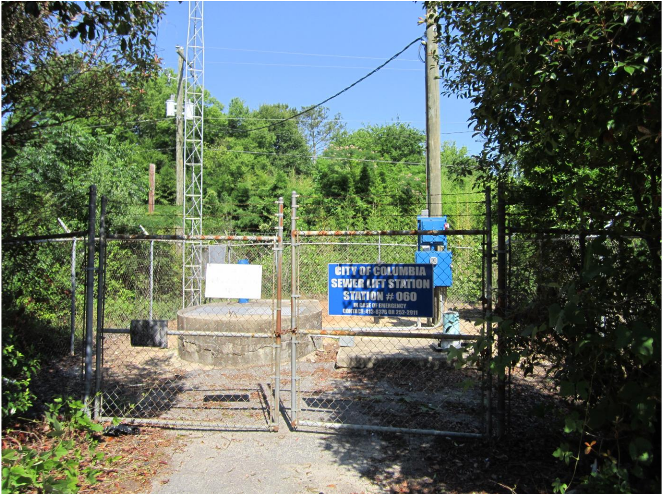
PHOTO 1: OVERALL PUMP STATION AND SITE ENTRANCE
