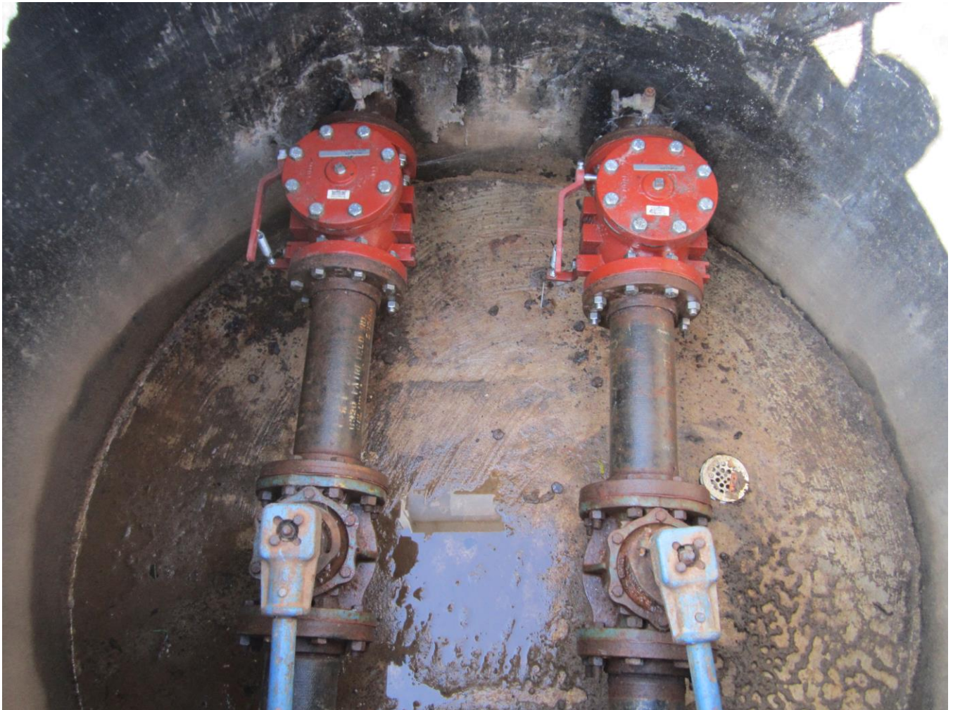
PHOTO 2: DISCHARGE HEADER
