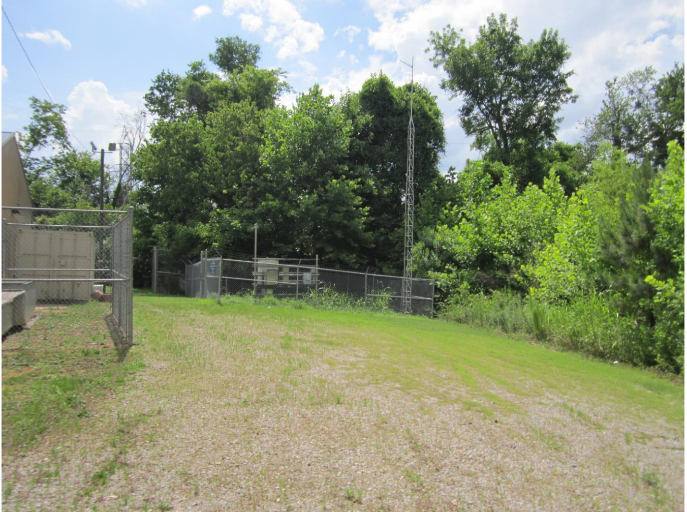
PHOTO 1: OVERALL PUMP STATION SITE
