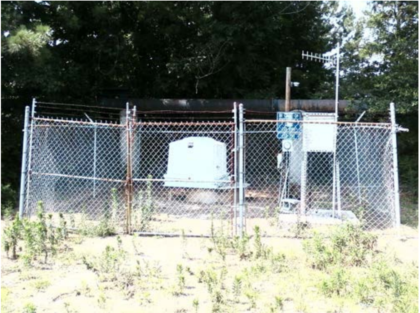
PHOTO 1: OVERALL PUMP STATION SITE AND ENTRANCE
