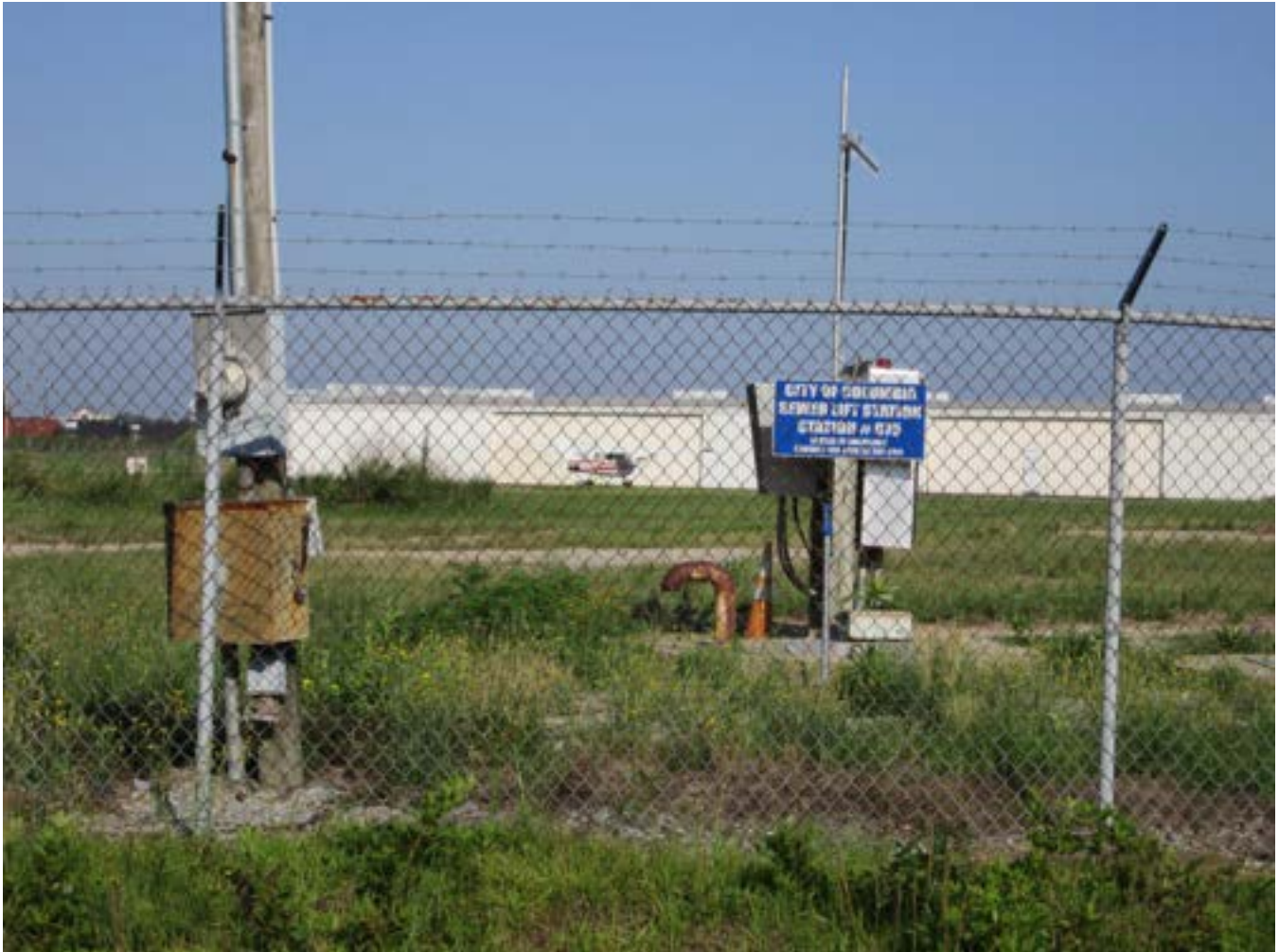
PHOTO 1: OVERALL PUMP STATION SITE
