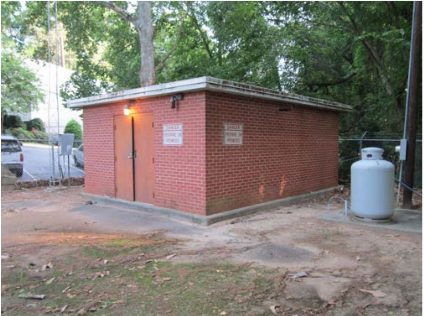
PHOTO 1: OVERALL PUMP STATION SITE
