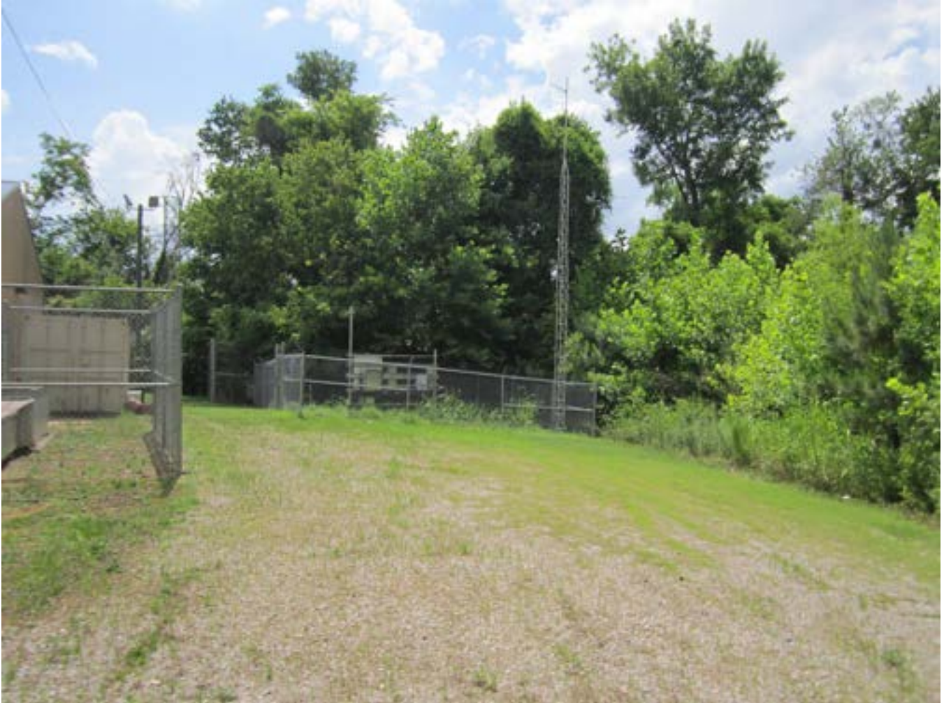
PHOTO 1: OVERALL PUMP STATION SITE
