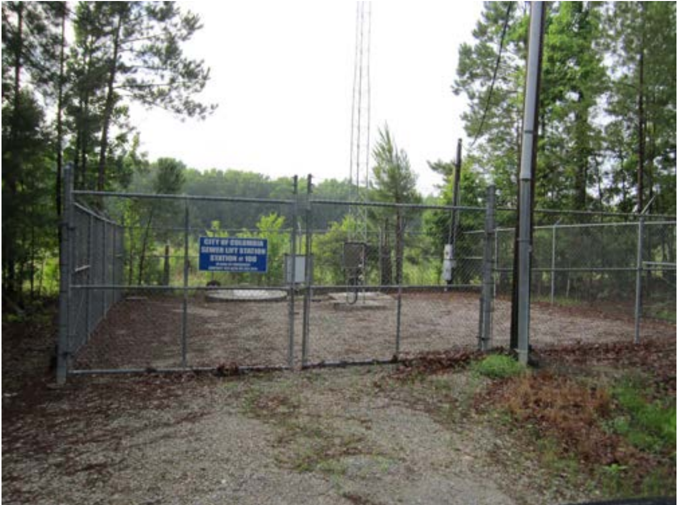
PHOTO 1: OVERALL PUMP STATION AND SITE ENTRANCE
