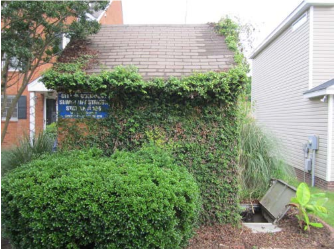
PHOTO 1: PUMP STATION EXTERIOR
