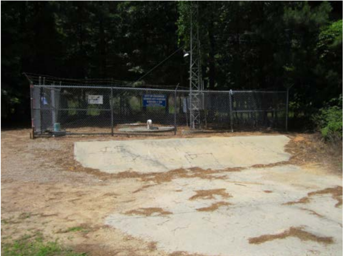
PHOTO 1: OVERALL PUMP STATION SITE AND ENTRANCE
