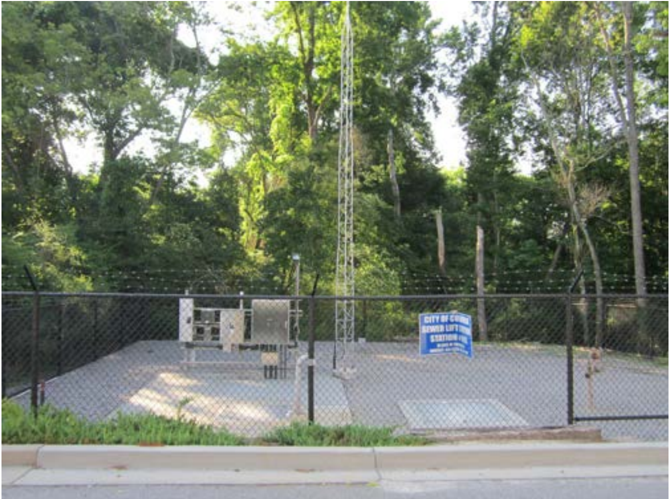
PHOTO 1: OVERALL PUMP STATION AND SITE ENTRANCE
