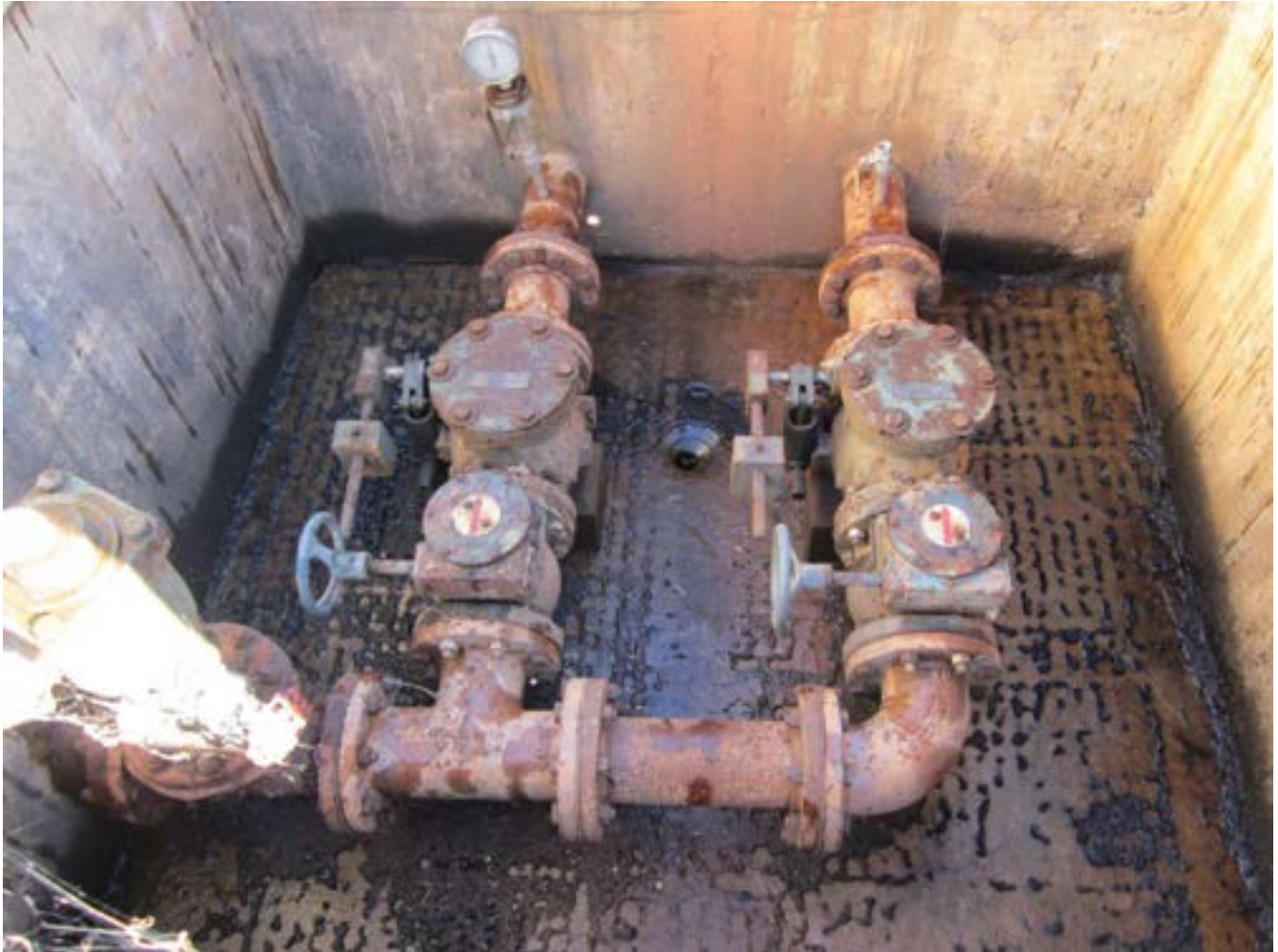
PHOTO 2: VALVE VAULT PIPING AND PRESSURE GAUGE
