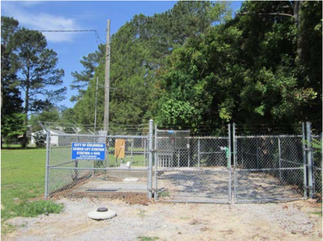
PHOTO 1: OVERALL PUMP STATION AND SITE ENTRANCE
