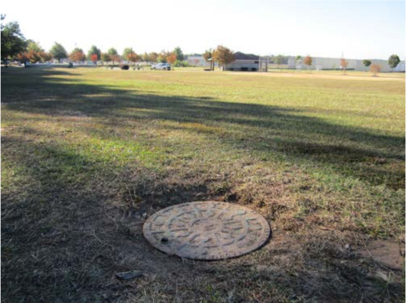
PHOTO 2: DISCHARGE MANHOLE AND PUMP STATION IN BACKGROUND
