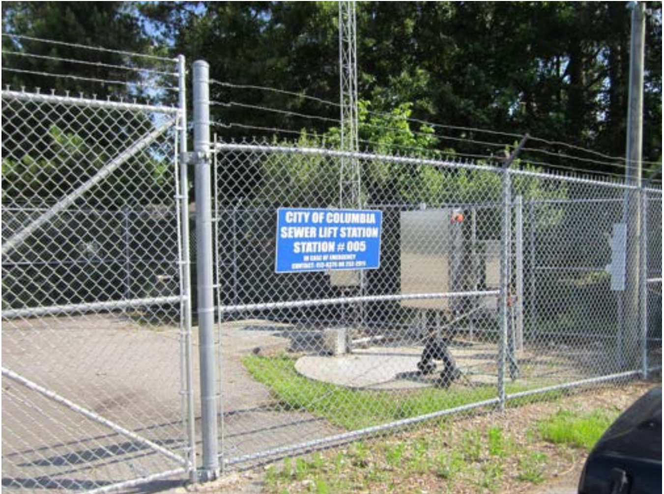
PHOTO 1: OVERALL PUMP STATION AND SITE ENTRANCE
