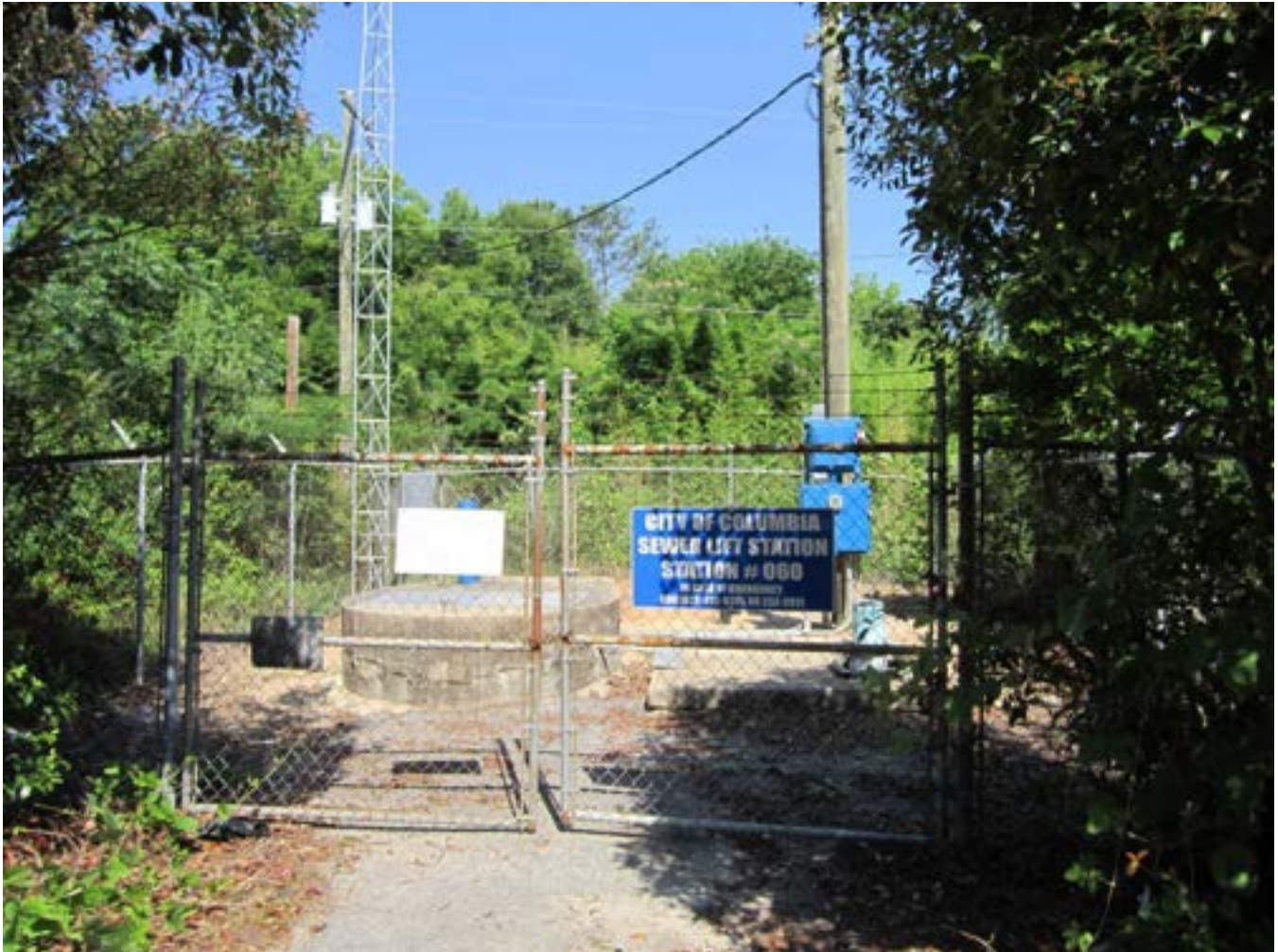
PHOTO 1: OVERALL PUMP STATION AND SITE ENTRANCE
