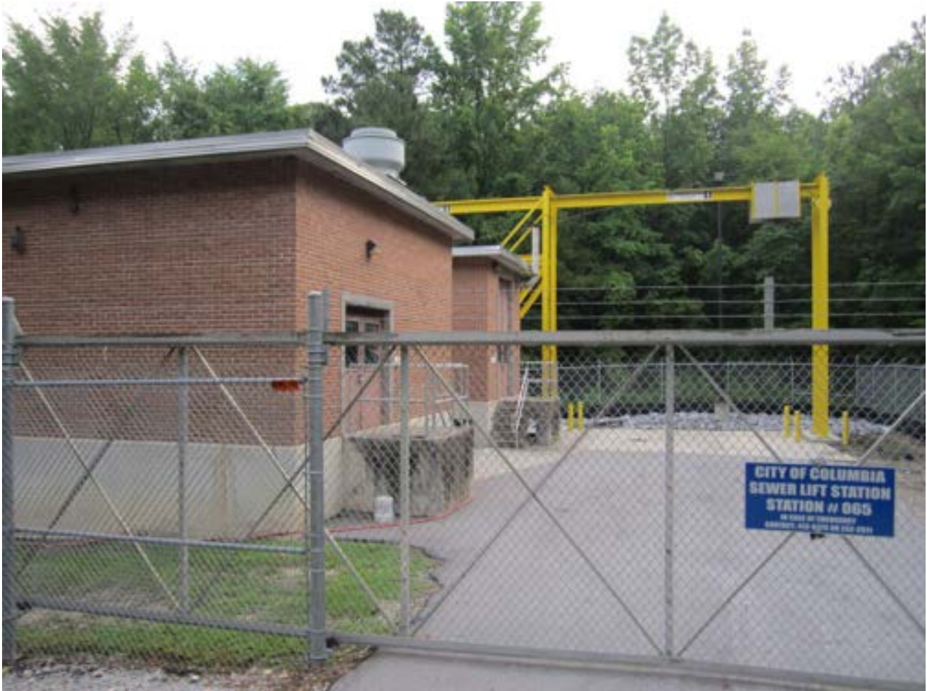
PHOTO 1: OVERALL PUMP STATION AND SITE ENTRANCE
