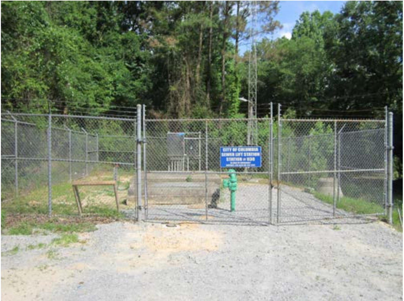
PHOTO 1: OVERALL PUMP STATION AND SITE ENTRANCE
