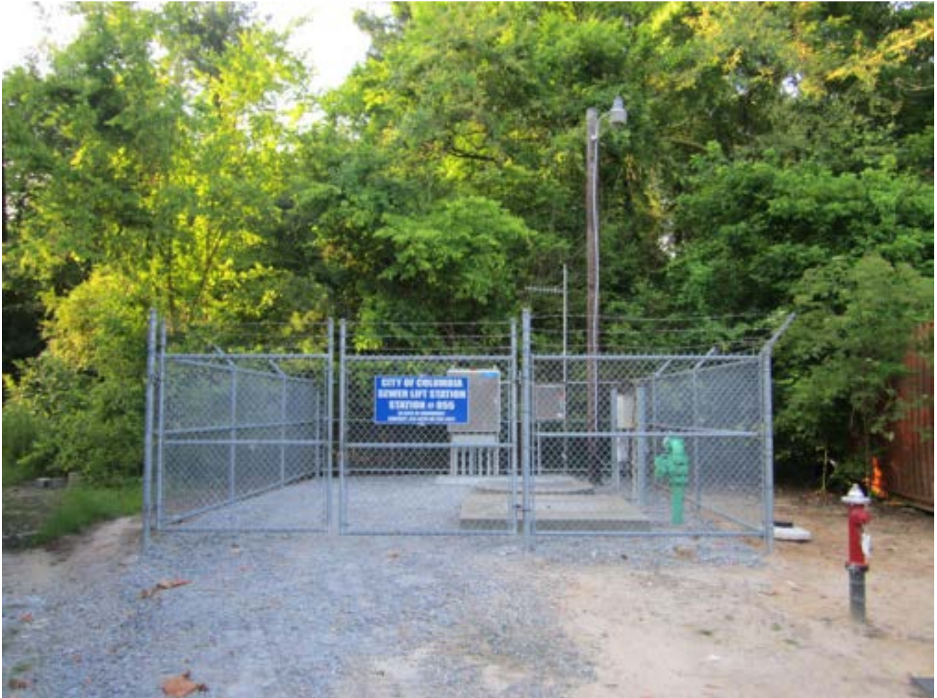
PHOTO 1: OVERALL PUMP STATION AND SITE ENTRANCE
