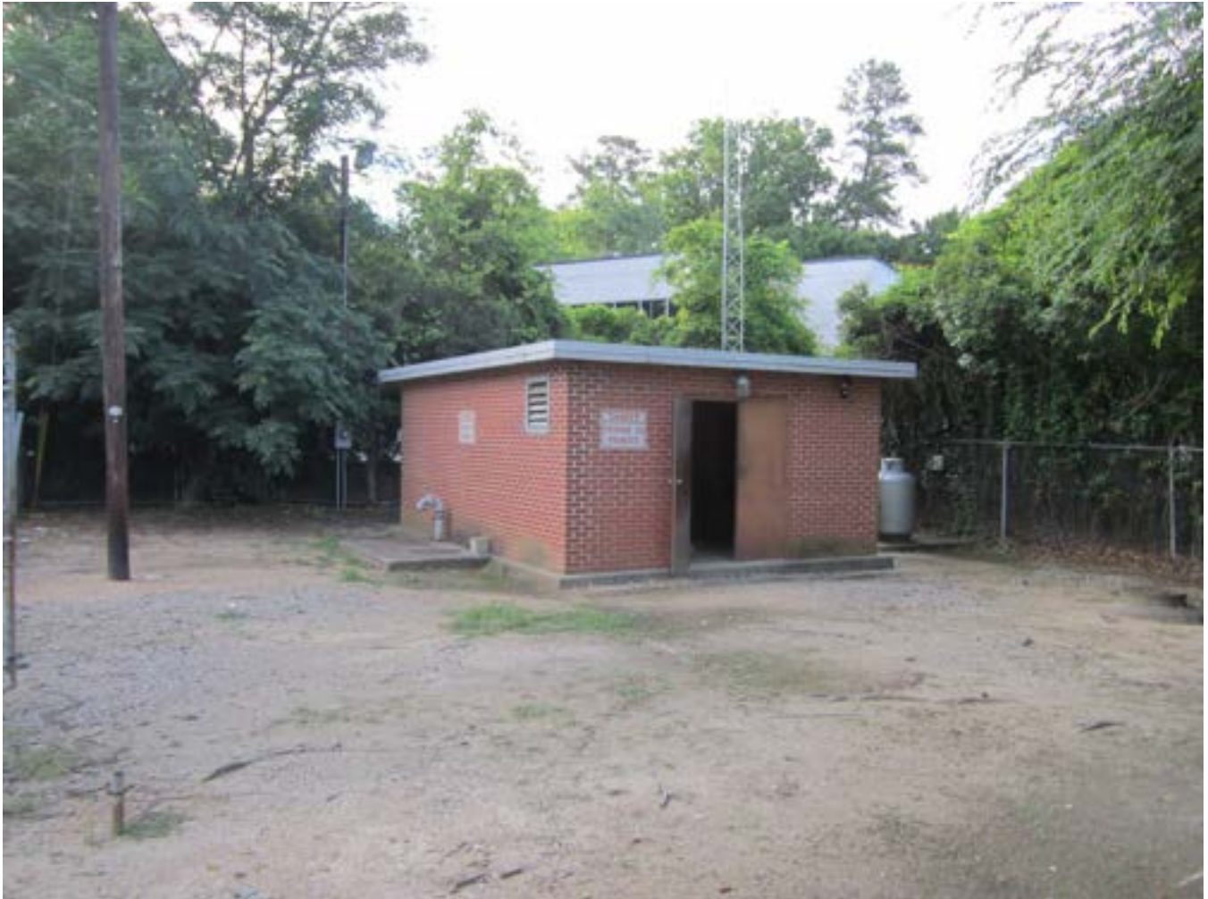
PHOTO 1: OVERALL PUMP STATION SITE AND ENTRANCE
