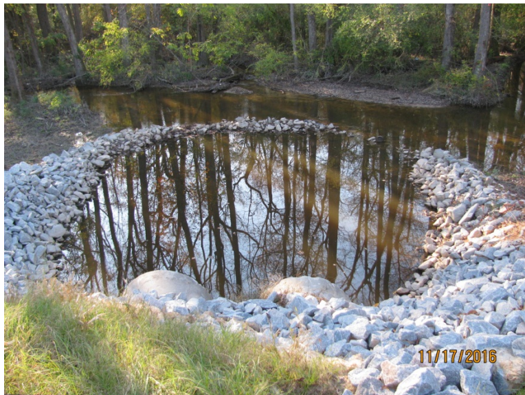
Riprap plunge pool at Site 4C
