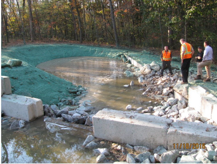
View of the third pool, facing downstream.
