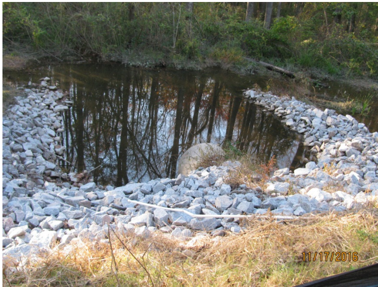
Riprap plunge pool at Site 4B
