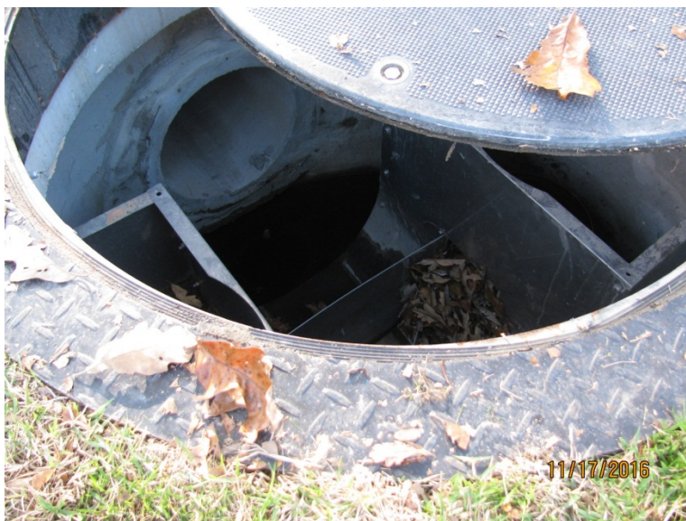
Interior view of the Site 6 MTD
