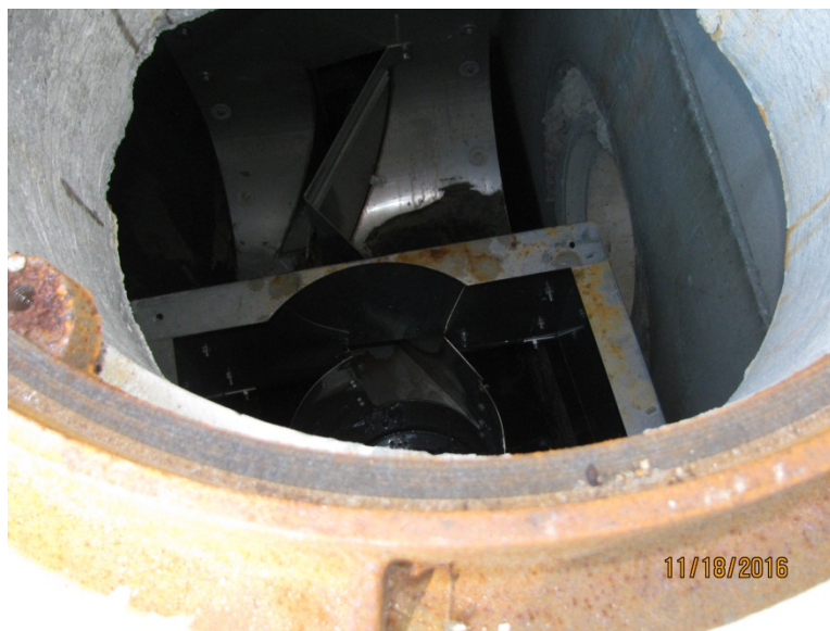
Interior view of Site 3 MTD
