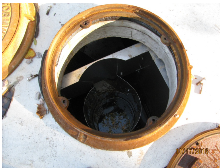
Interior view of the Site 1 MTD
