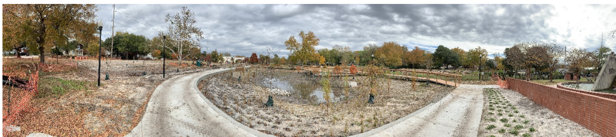
Panoramic picture of the park in December 2018 after major construction and the installation of the plantings and vegetation was completed.
