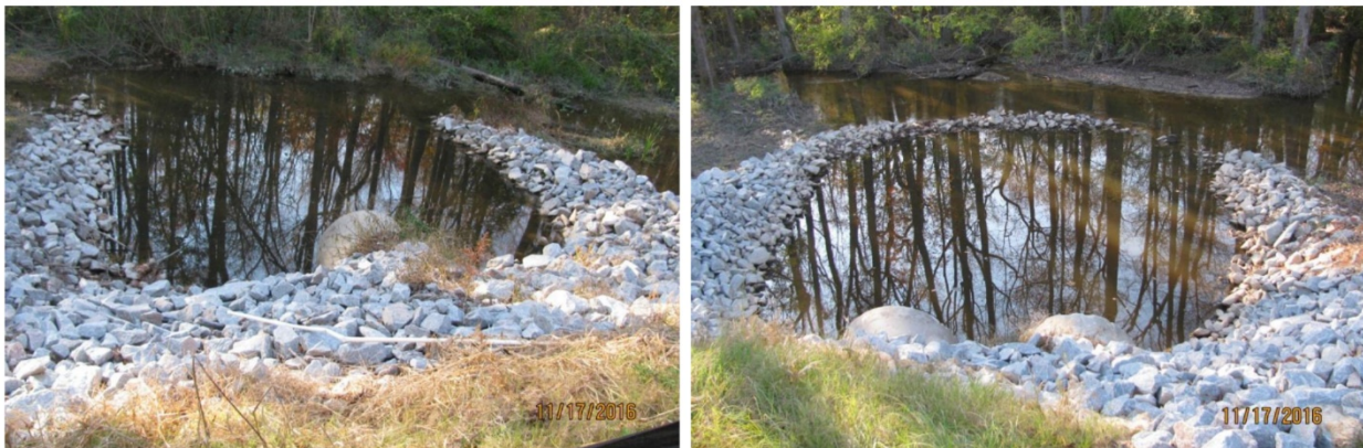
Riprap plunge pool at Site 4B (left) and 4C (right).
