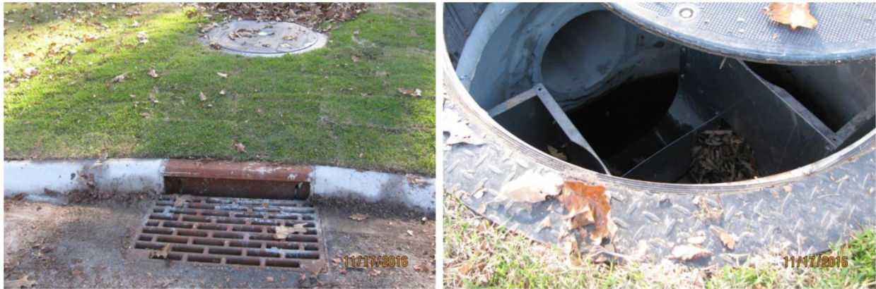
Surface view (left) and interior view (right) of the Site 6 MTD.
