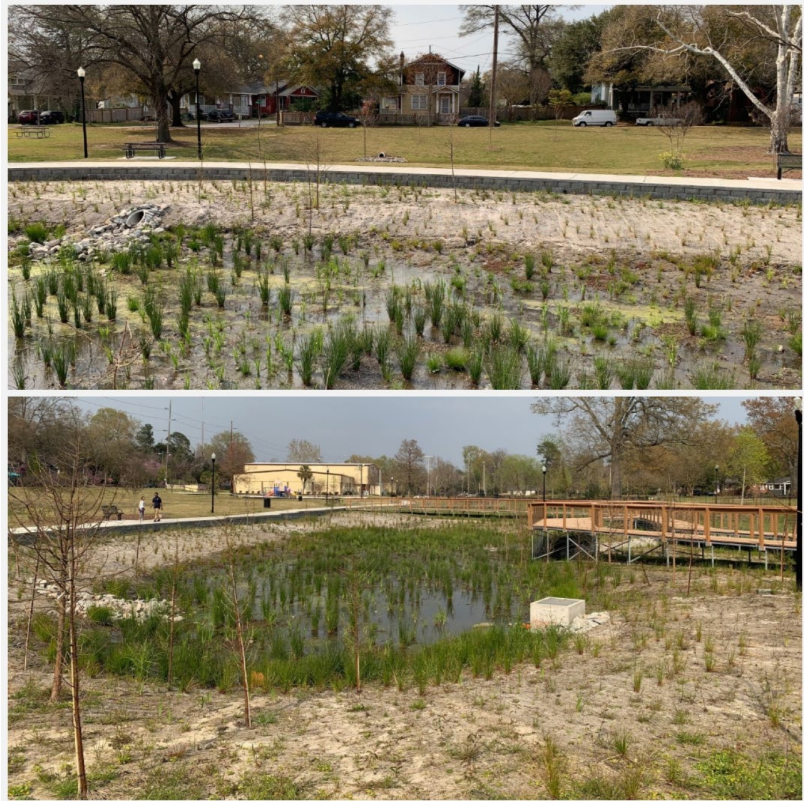
Two of the three detention areas (top) on site from March 2019. Flow from the smaller detention area (top of the picture) enters the larger detention area through the detention pond inlet shown; picture of the large detention area and boardwalk from March 2019.
