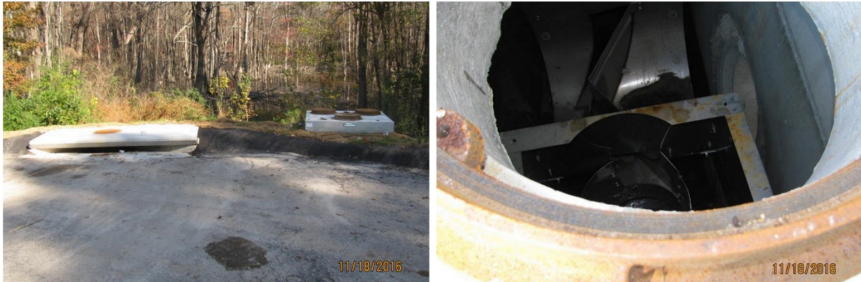
Surface view (left) and interior view (right) of Site 3 MTD and inlet.
