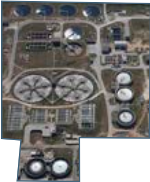
Treatment Train #1 40 MGD
