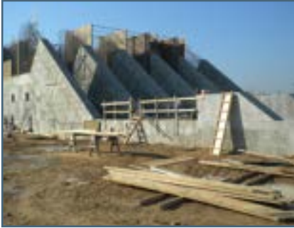
Construction of the new headworks facility at the Metro WWTW
